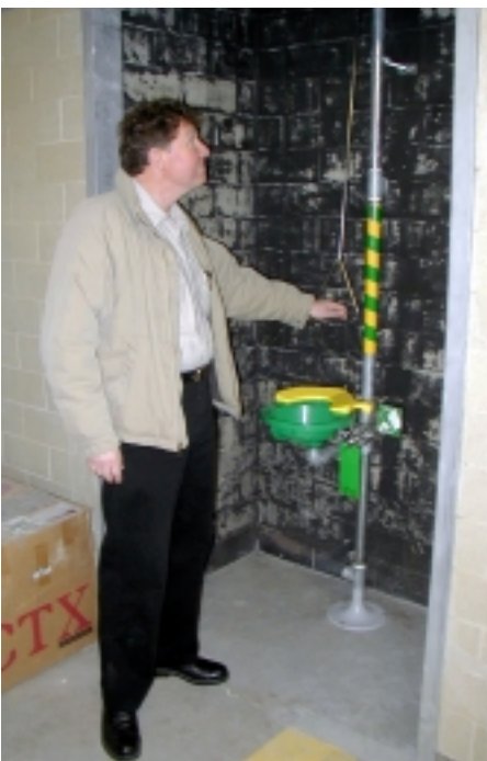
Rich Cutler points out one of the new safety stations that will eventually be installed on every floor of all lab buildings.
